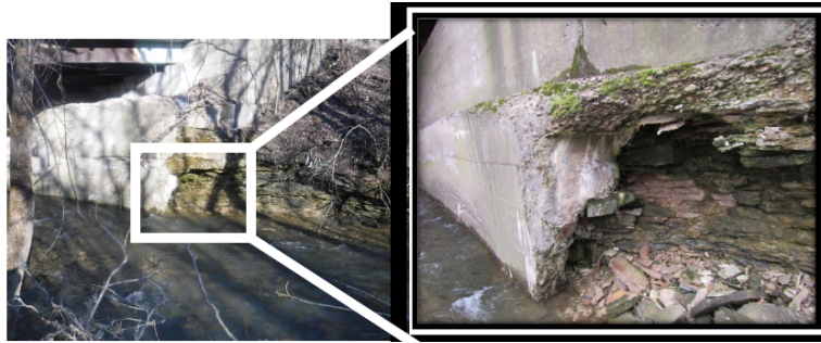
Figure 5 Bridge with non-scour-resistant rock.
