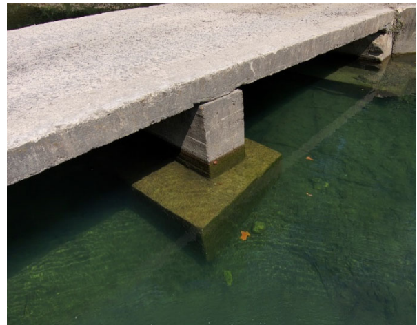
Figure 2 Exposed footing with undermining.
