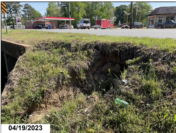
Bent 1 left has slope erosion.
