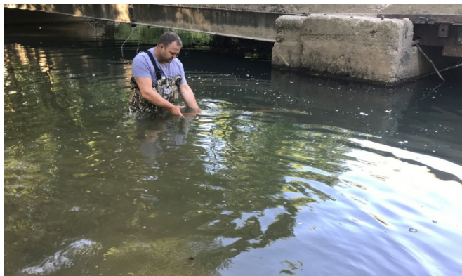
Figure 3 Wading and Probing.
