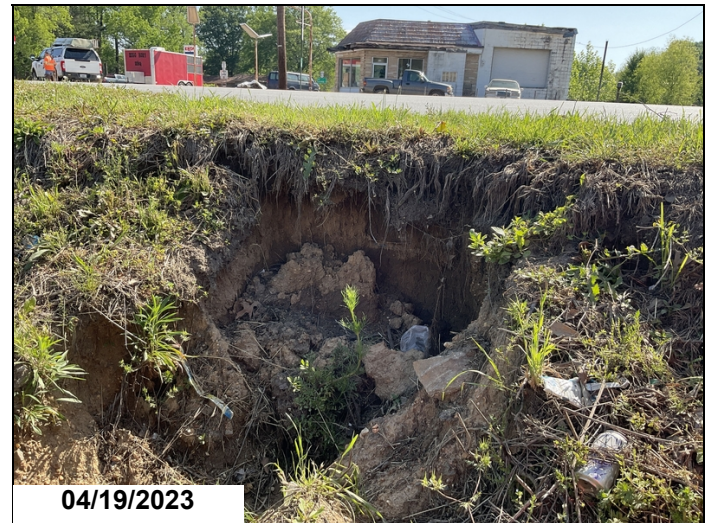
Bent 1 left side slope erosion.
