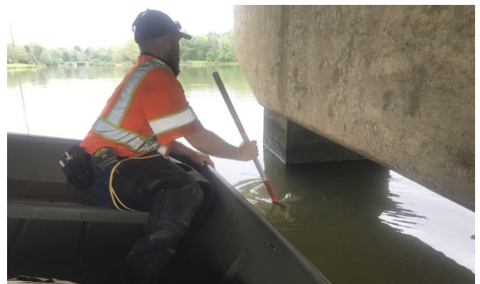
Figure 4 Probing from a boat.
