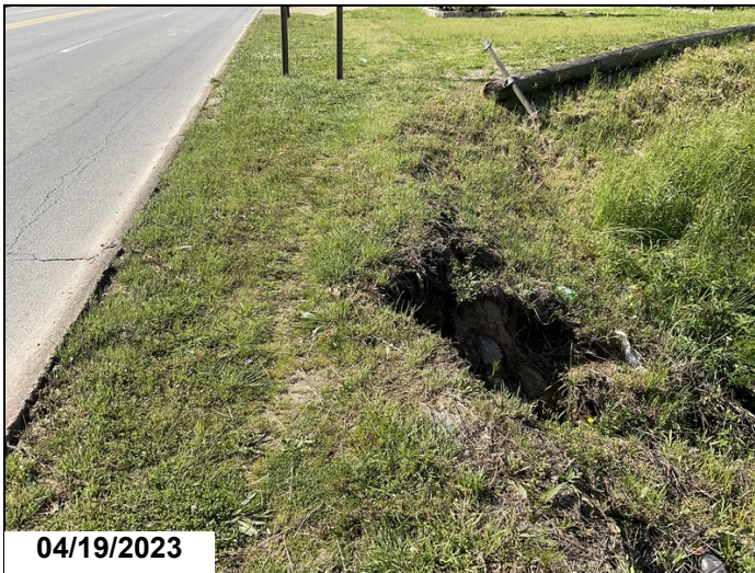
Bent 1 left side slope erosion.
